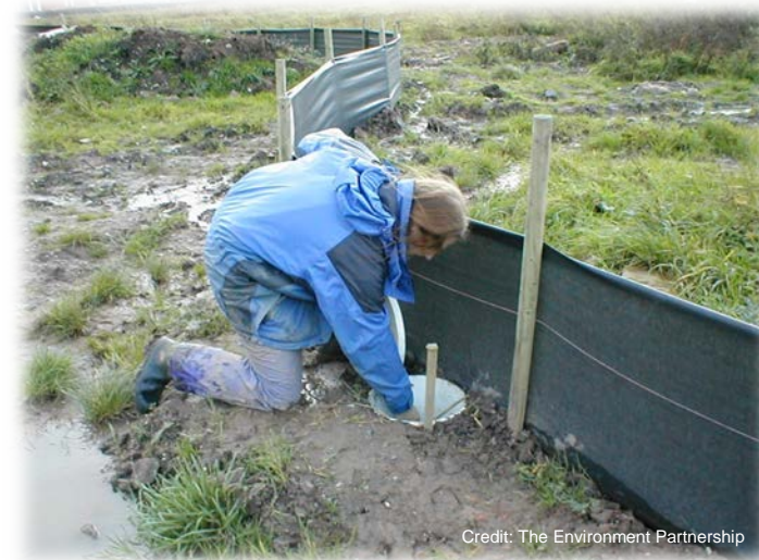
Figure B5.3: Newt exclusion fencing and capture of newts from development sites within 500m of a breeding GCN pond prior to development commencing is a common mitigation measure.
